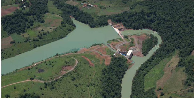
Aerial view of the Rodeio Bonito plant
